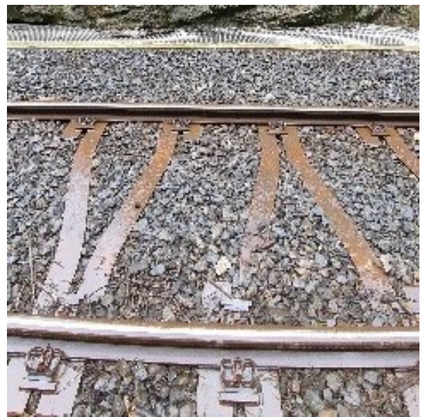
Figure 3.30 – Harrachov Locality – Position of a Thermometer in the Rock Cutting (Thermometer from the bottom of the Rail Foot), Author Dr. Vladimír Suchánek
