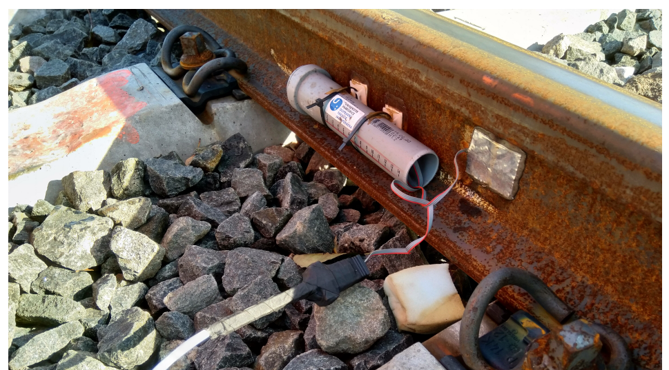
Figure 4: Connection of track and mobile part of the measuring set during measurement.
