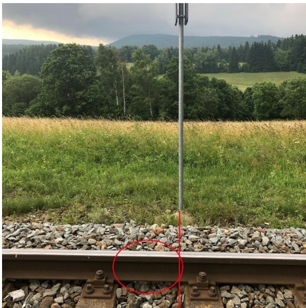
Figure 3.17 – Ostružná Locality – Position of a Thermometer on the Rail Bridge (Thermometer from the bottom of the Rail Foot), Author Miloš Šula
