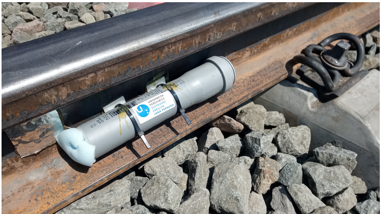
Figure 4.13 – Measuring Set Track Unit
