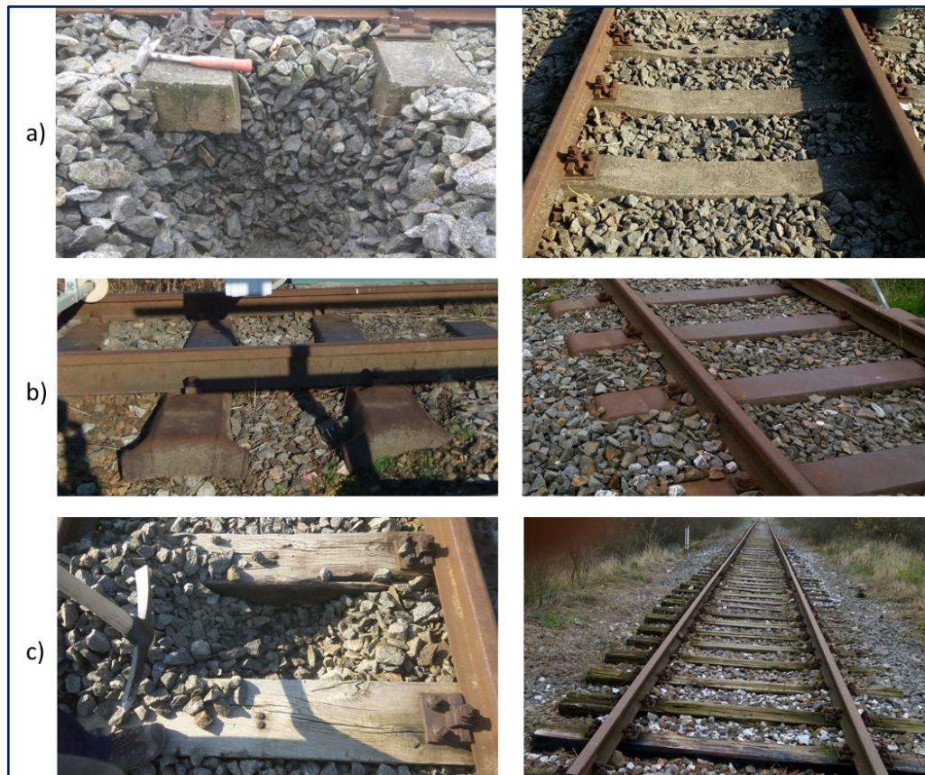
Figure 1.5. Sleeper types according to the material it is made of a) reinforced concrete, b) steel, c) wooden
