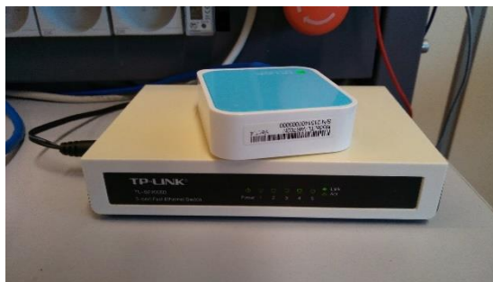
Obr. 6.2 – Router a switch
