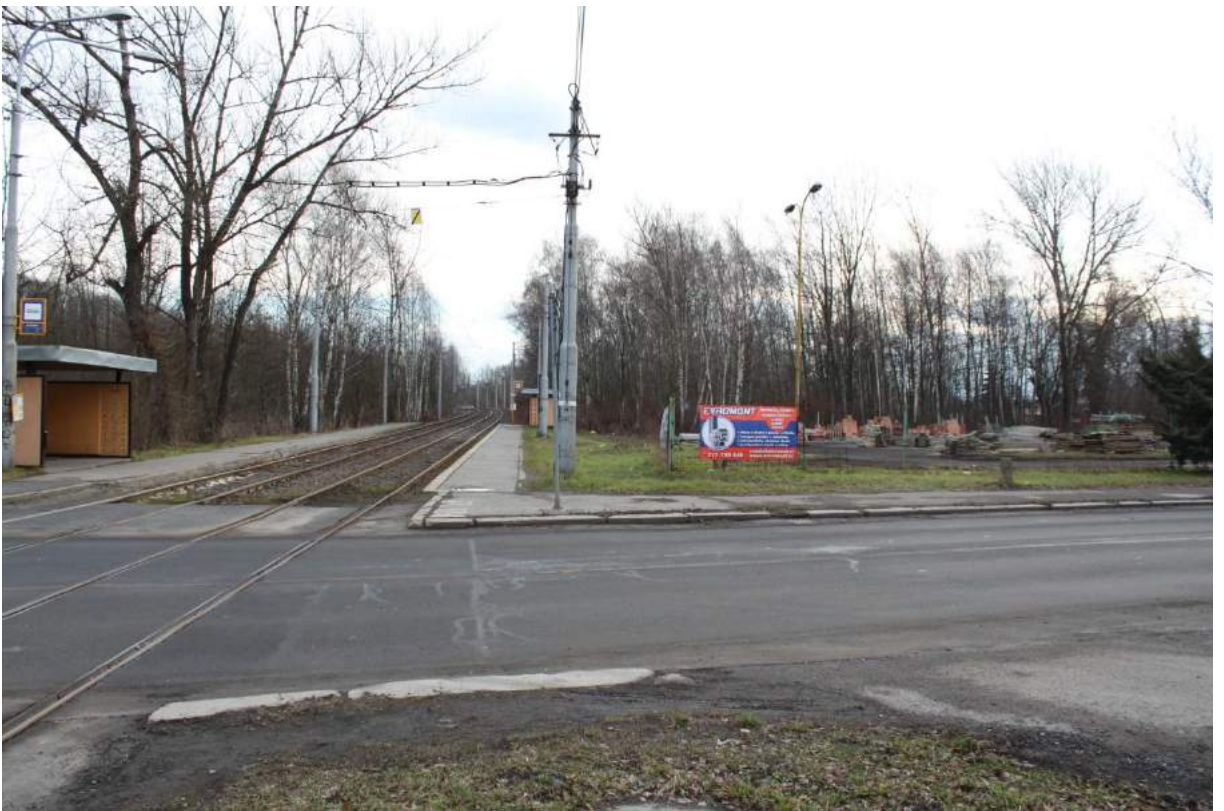
Figure 25 - Tram stop "Důl Zárubek" with an area of former railway yard
