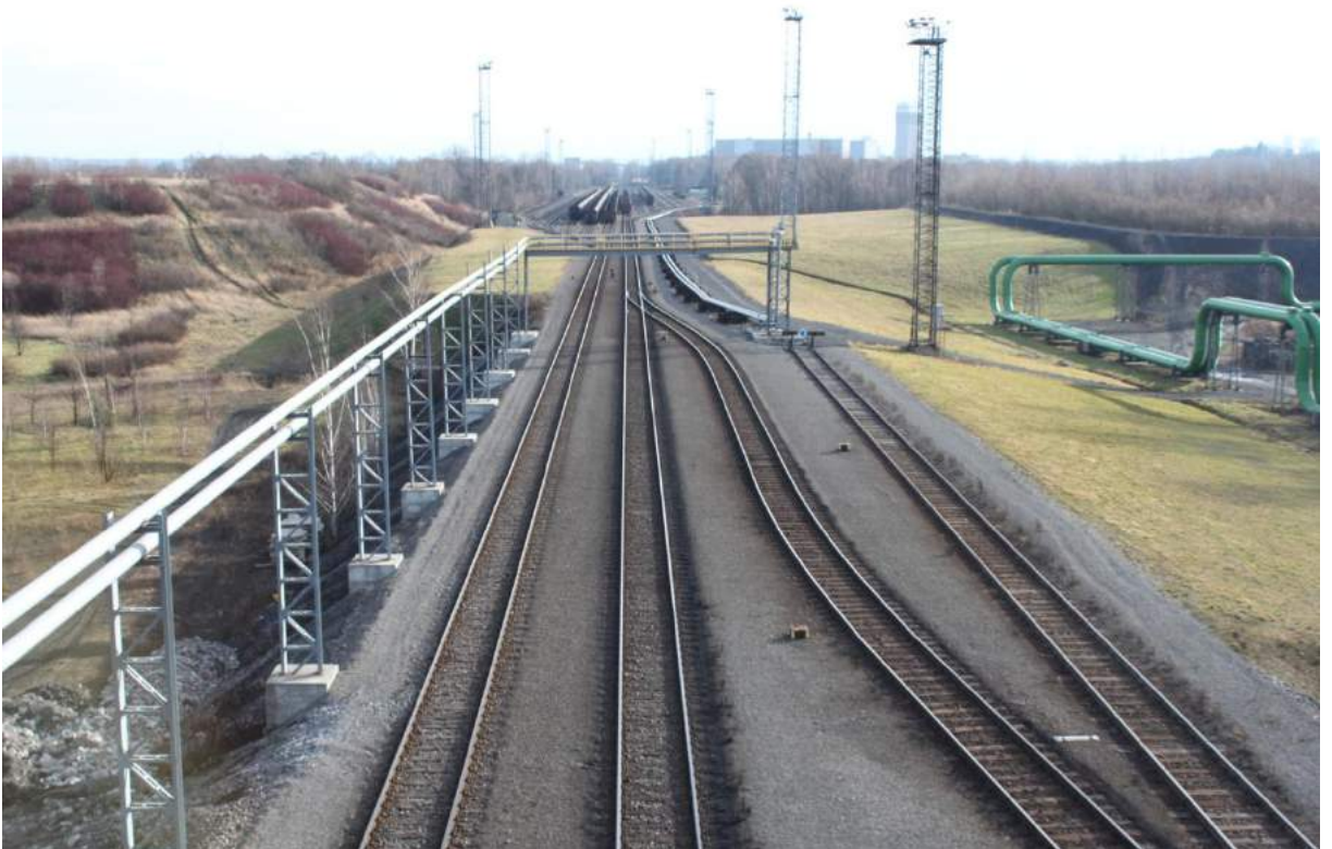
Figure 32 - The old railway station of the city of Karviná
