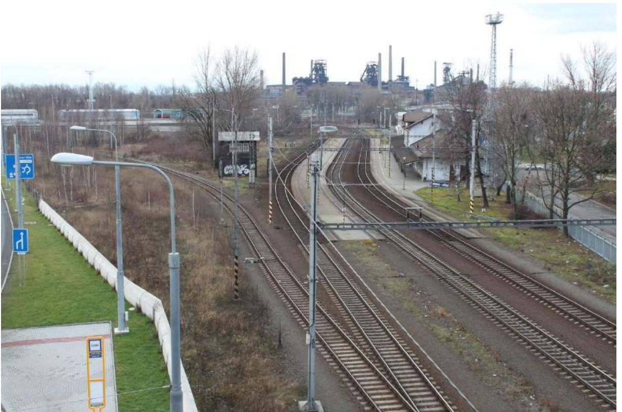
Figure 27 - A general view of Ostrava střed station
