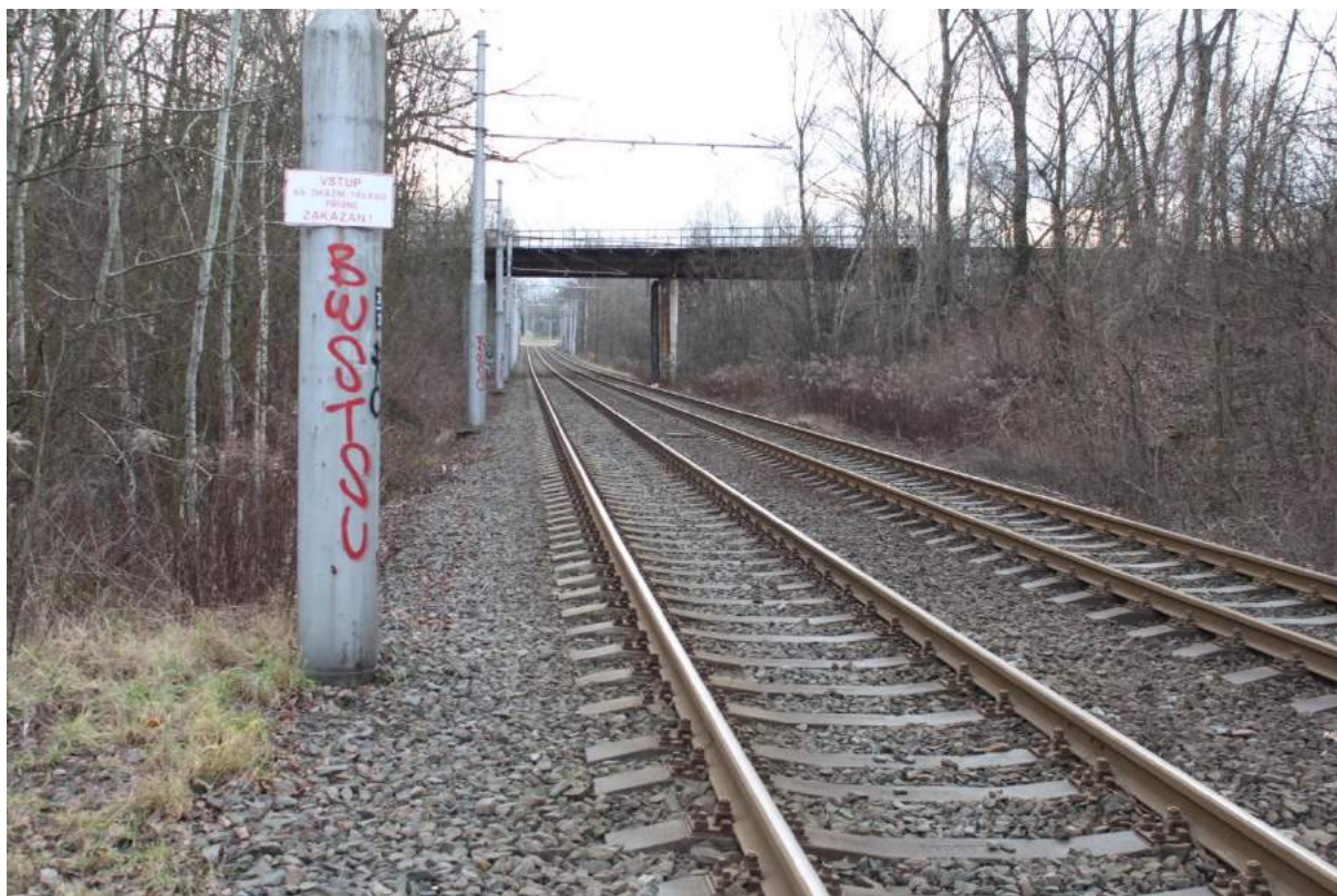
Figure 18 - A view of the proposed Hranečník junction; tram tracks in the foreground, designed train-tram line bridge in the background; the connecting track is supposed to be in the wood on the left side
