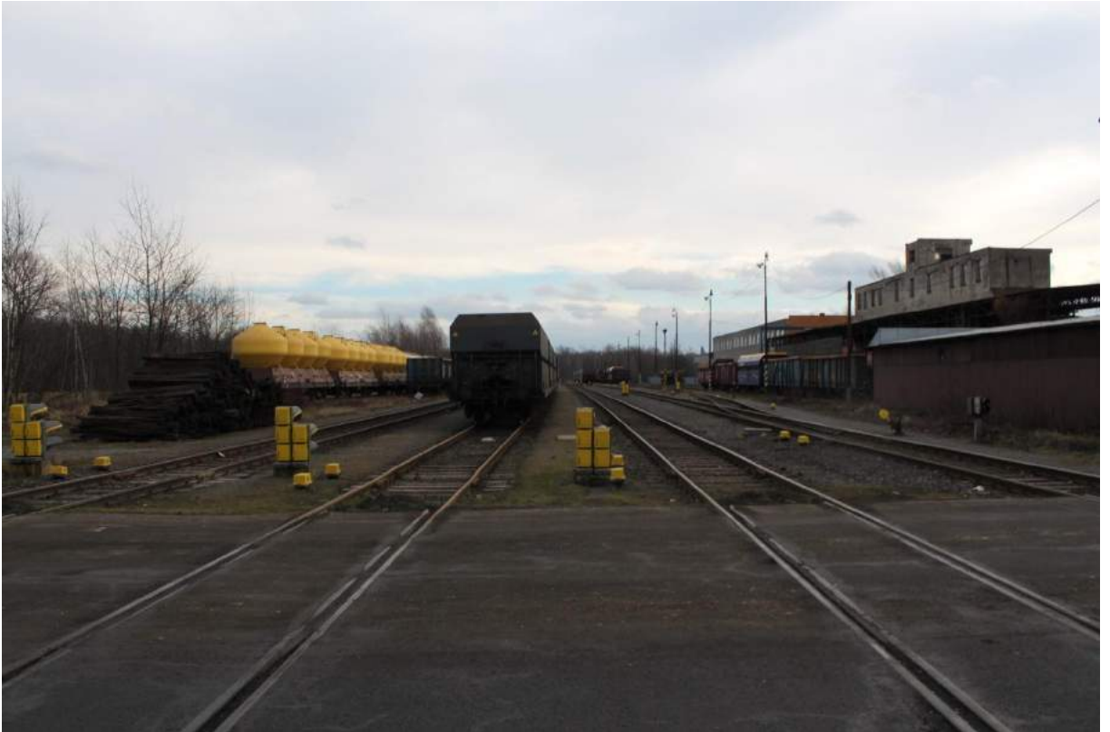
Figure 26 - Railway yard at Důl Zárubek coal mine
