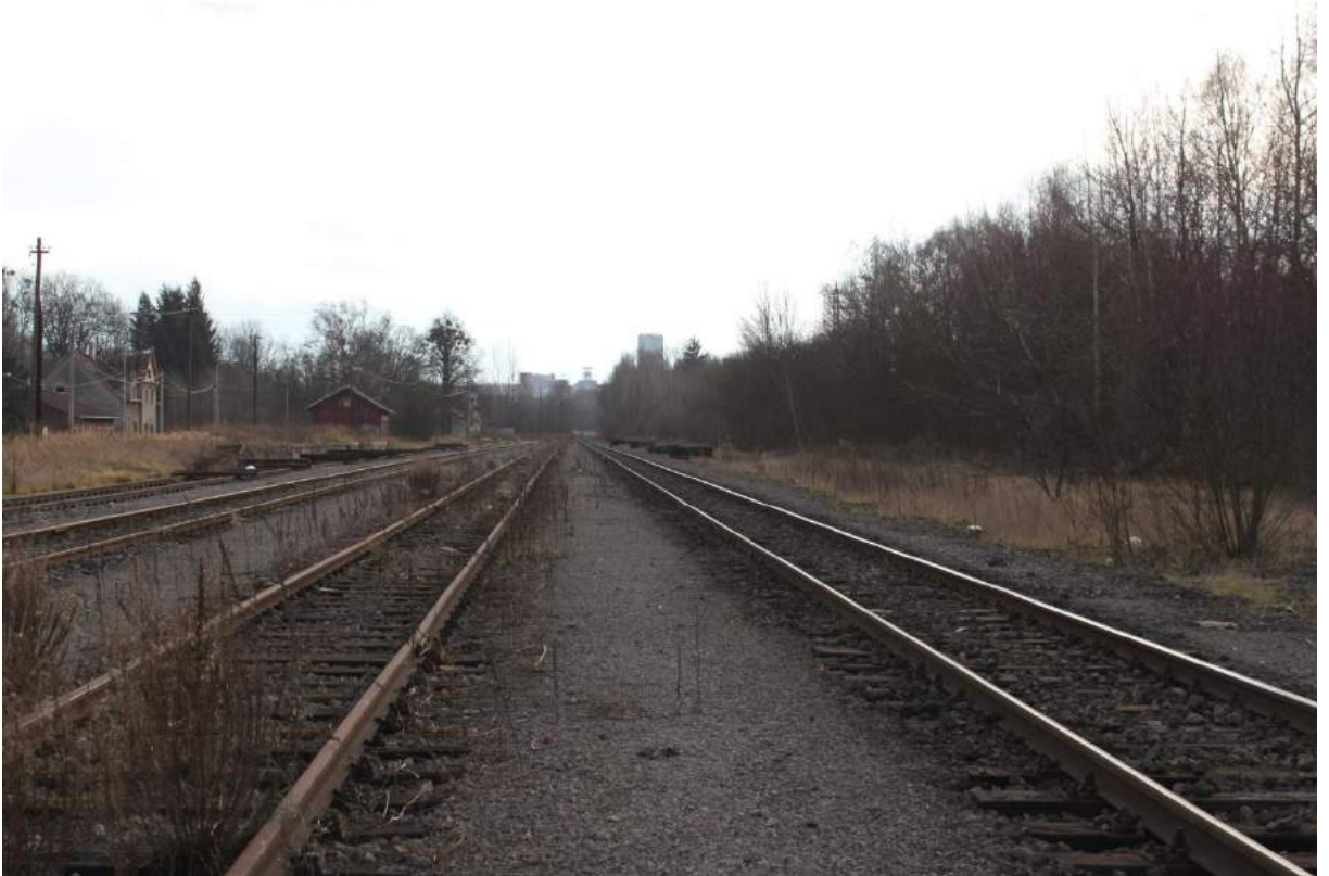
Figure 31 - Railway station Orlová
