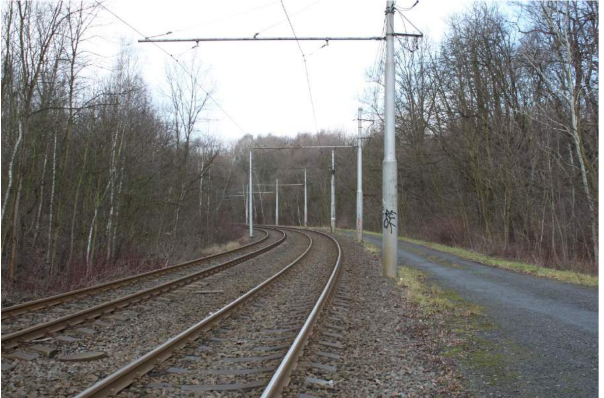
Figure 24 - Tram track section Černá louka - Hranečník in Ostrava
