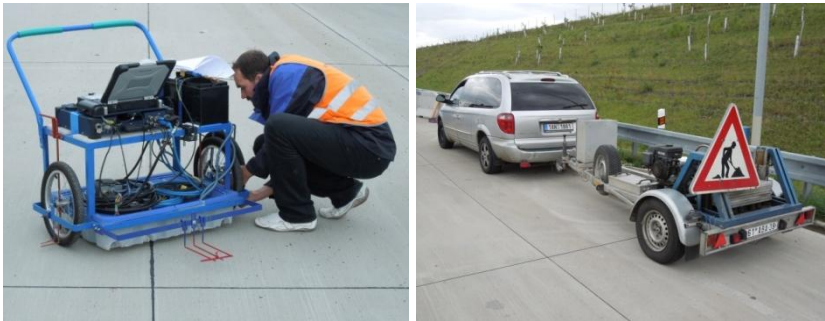
Fig. 6 Application of non-destructive methods for evaluation of dowels and tie bars positions on testing segments
