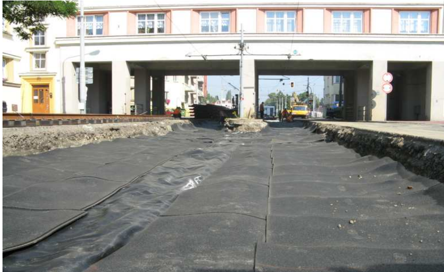
Fig.3: The installation of anti-vibration mats CONIRAP
