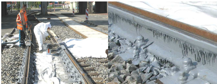
Fig.4: Spray rails and consolidator polyurethane CONUPUR M800
